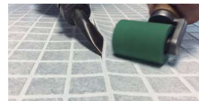
Butt welded seams
