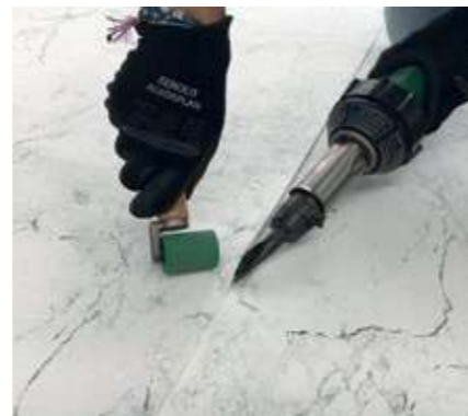
2 nd Welding on the outside of the overlap
